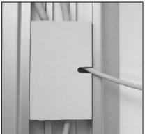
**8.2** Press one side of the Cover into channel, routing cables behind Cover and through notches. Squeeze Cover and insert other side into channel.
